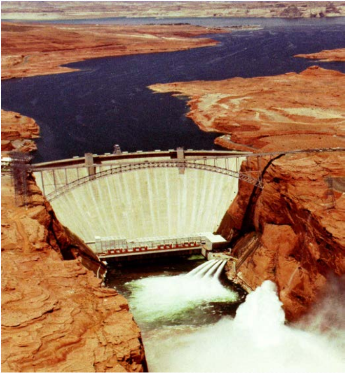
The Glen Canyon Dam on the Colorado River in Arizona, United States.
